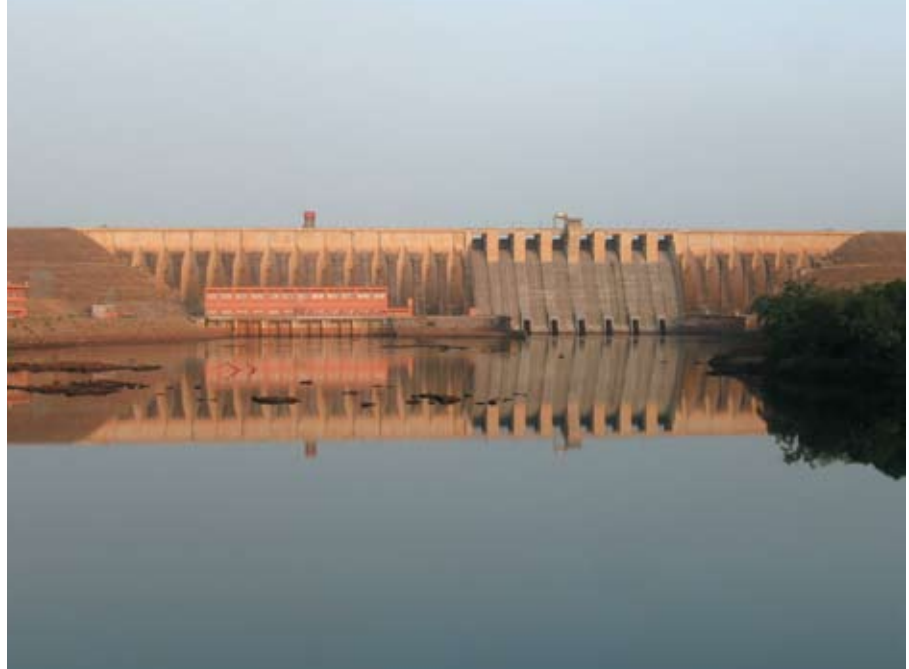
Manantali Dam on the Senegal River.
