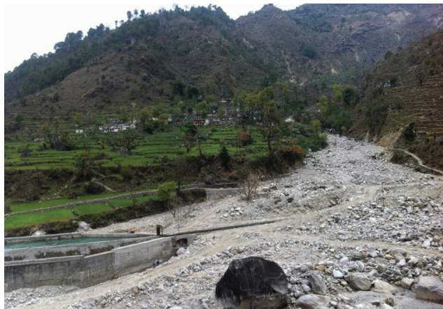
Dry riverbed on India’s Nandakini River, whose flows are diverted through a series of tunnels.
