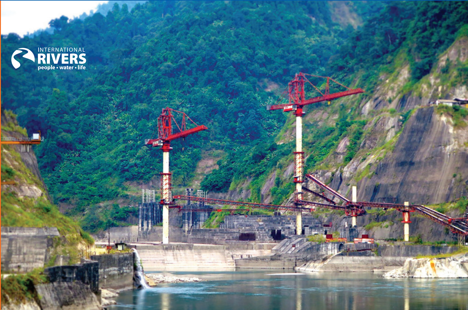
Lower Subansiri Dam, India. Credit: Keith Schneider, Circle of Blue
