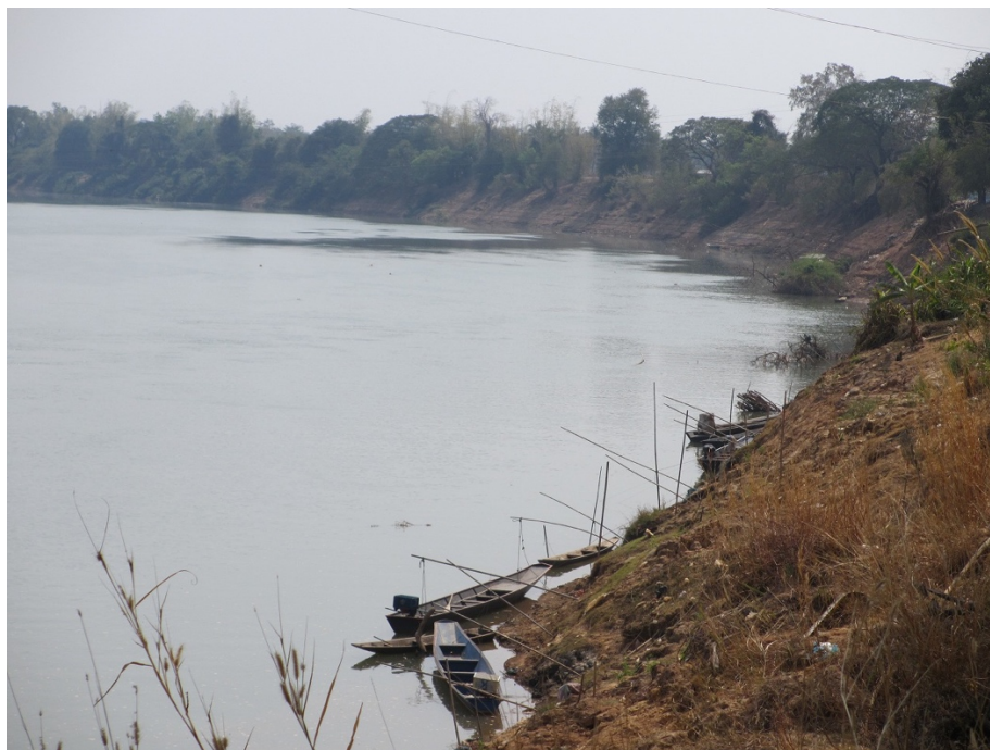
Xe Bang Fai – Riverbank erosion in Boua Khai village (Photo credit: Mekong Watch)
