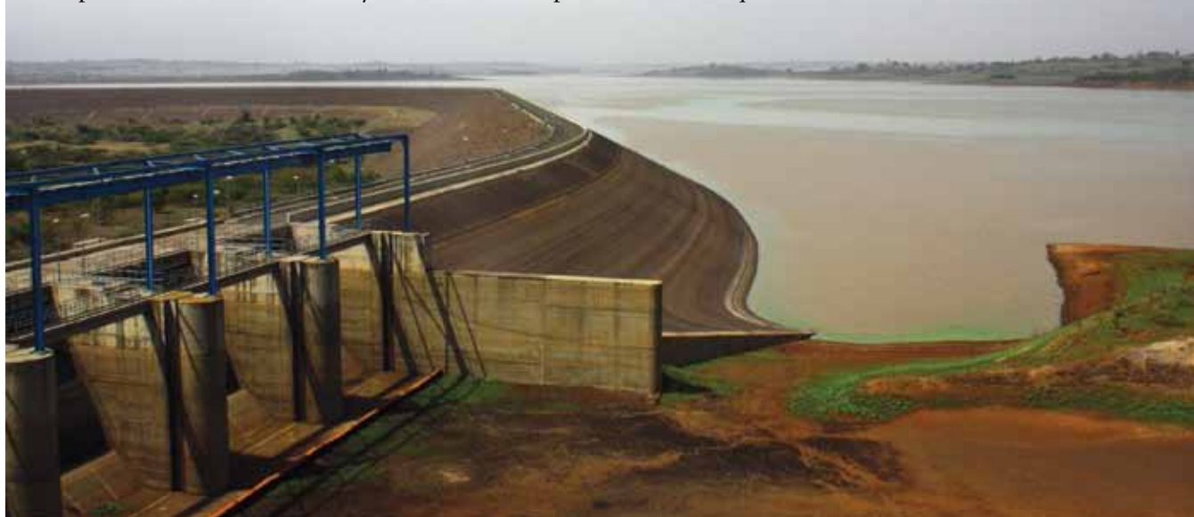
Construction of the Gibe 3 dam. Photo: FIVAS, Jarand Ullestad
