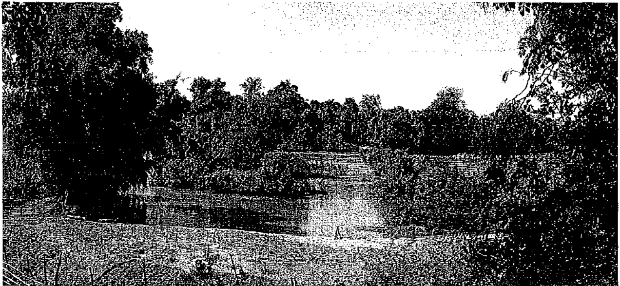
Photo 12.1 – View across Hou Sahong above Upstream Cofferdam Site (River flows right to left)
