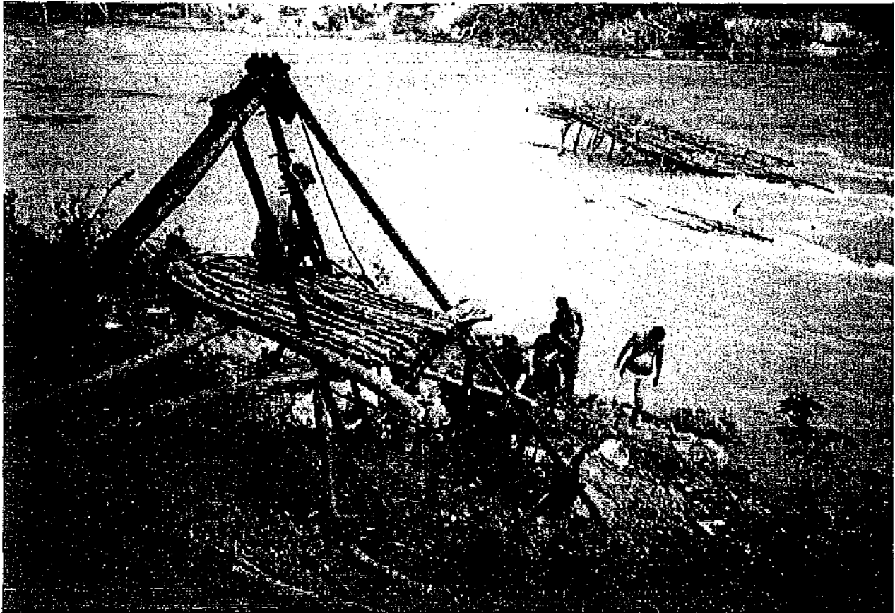
Photograph 5-3 ~ Inclined Borehole BL14, left bank, near lower dam site axis.
