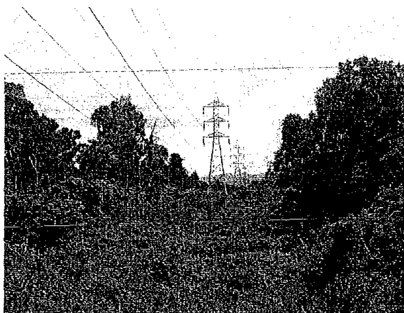
Photo 9-5 - Double circuit transmission line between JiangXai and Ban Na
