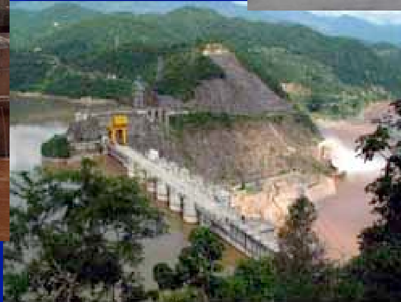
The backside of Manwan dam
