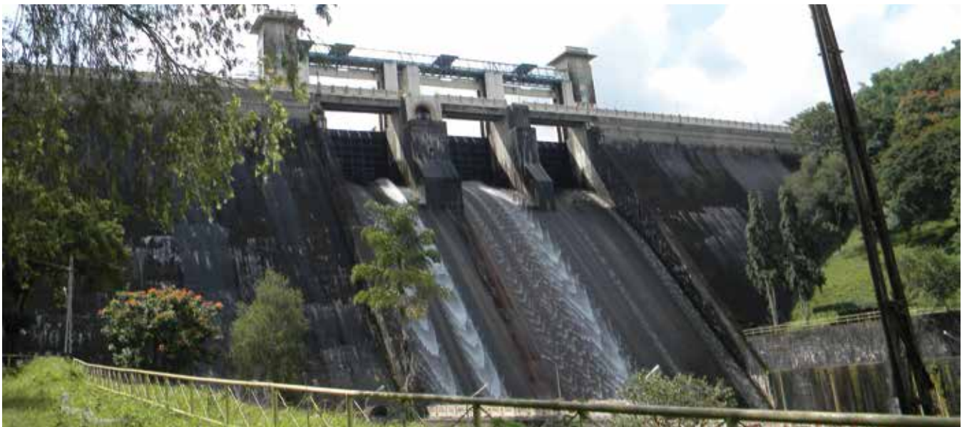
Parambikulam Dam. Photo credit: Latha Anantha
